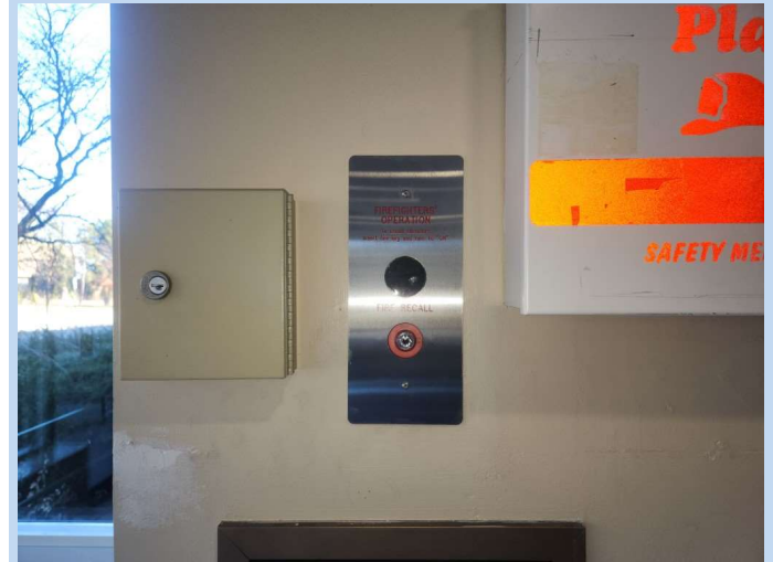
The auxiliary fire key switch in the front vestibule.
