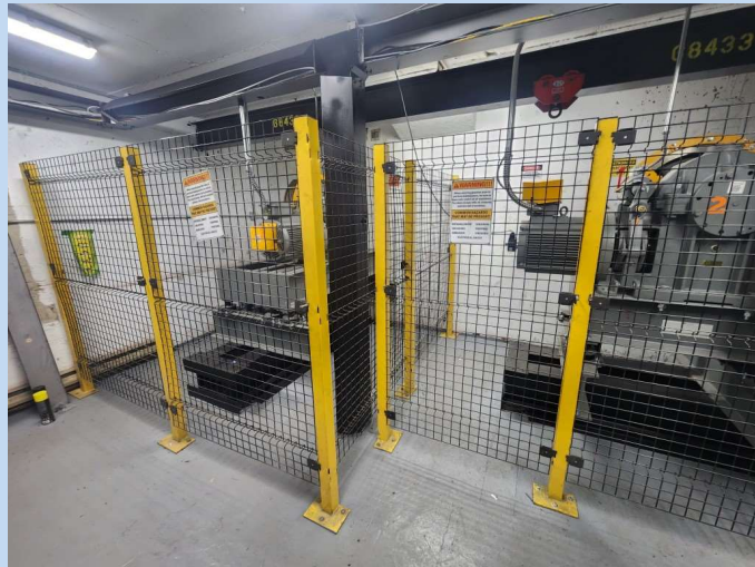
The elevator machine room guarding installed and the floor painted.
