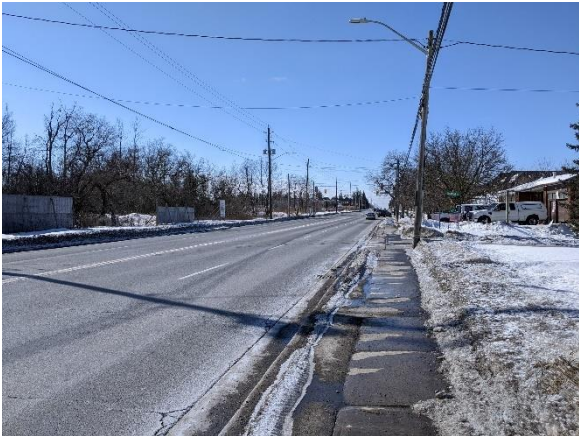
VIEW ALONG KIND RD, LOOKING WEST
