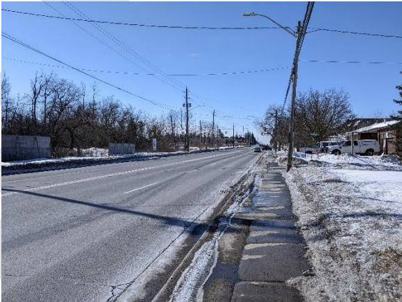
VIEW ALONG KIND RD, LOOKING WEST
