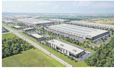
The rooftop solar panels at the James Snow Business Park in Milton, Ont., seen in a rendering, will generate power for tenants without them relying on the provincial grid all the time. OXFORD PROPERTIES
