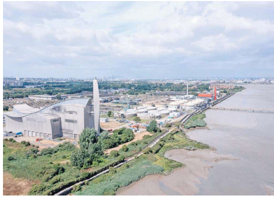
An aerial view shows Thames Water's Crossness Sewage Treatment Works on the banks of the River Thames in southeast London. The utility has been struggling under £14-billion of debt, aging infrastructure and widespread criticism about sewage spills and leaking pipes. BEN STANSALL/AFP VIA GETTY IMAGES
