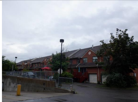
View of townhouse building rear
