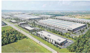
The rooftop solar panels at the James Snow Business Park in Milton, Ont., seen in a rendering, will generate power for tenants without them relying on the provincial grid all the time. OXFORD PROPERTIES
