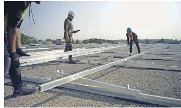
Rabba Fine Foods is currently installing solar panels on the roofs of two of the company's distribution warehouses. JOHN BREGGAR PHOTOGRAPHY
