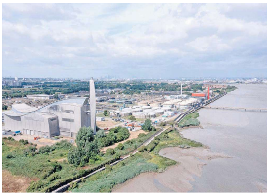
An aerial view shows Thames Water's Crossness Sewage Treatment Works on the banks of the River Thames in southeast London. The utility has been struggling under £14-billion of debt, aging infrastructure and widespread criticism about sewage spills and leaking pipes. BEN STANSALL/AFP VIA GETTY IMAGES
