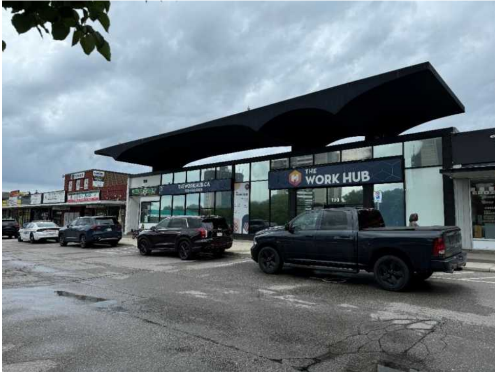
View of existing improvements
