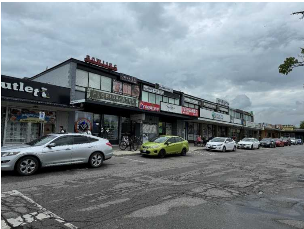
View of existing improvements
